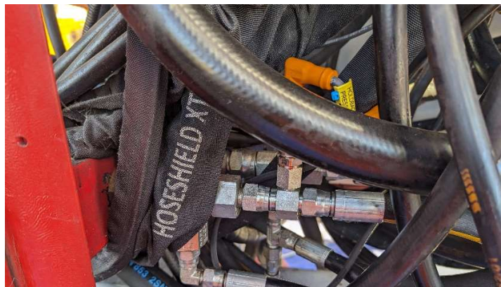
Figure 20 Pressure sensor location drivers side of control cab
