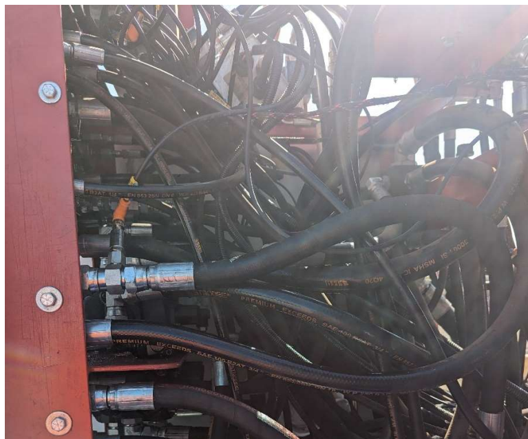
Figure 20 Rotation Pressure sensor location passengers side of control cab
