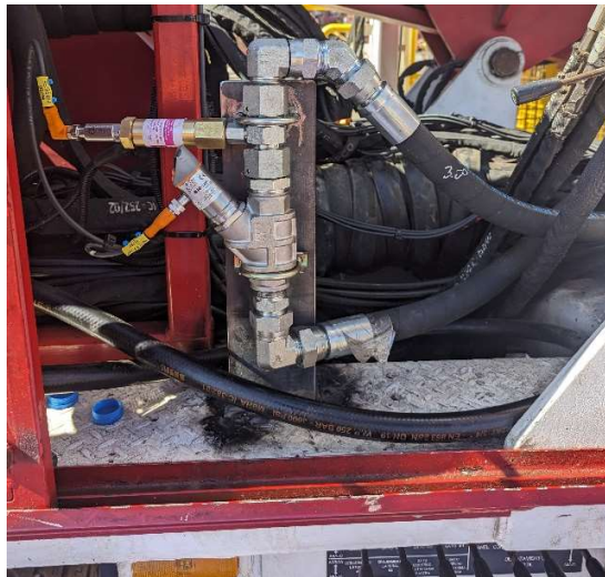
Figure 16 A12000 Water Flow and pressure Assembly
